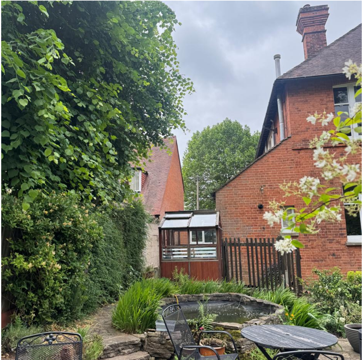
Figure 8: Rear of No. 73
