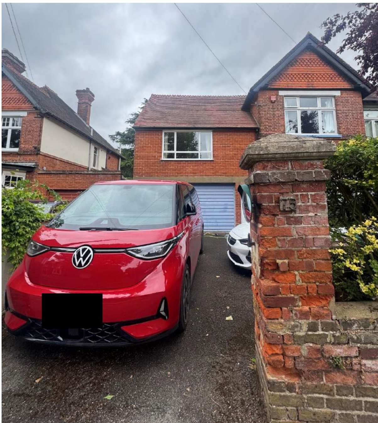
Figure 4: Front Elevation of No. 75
