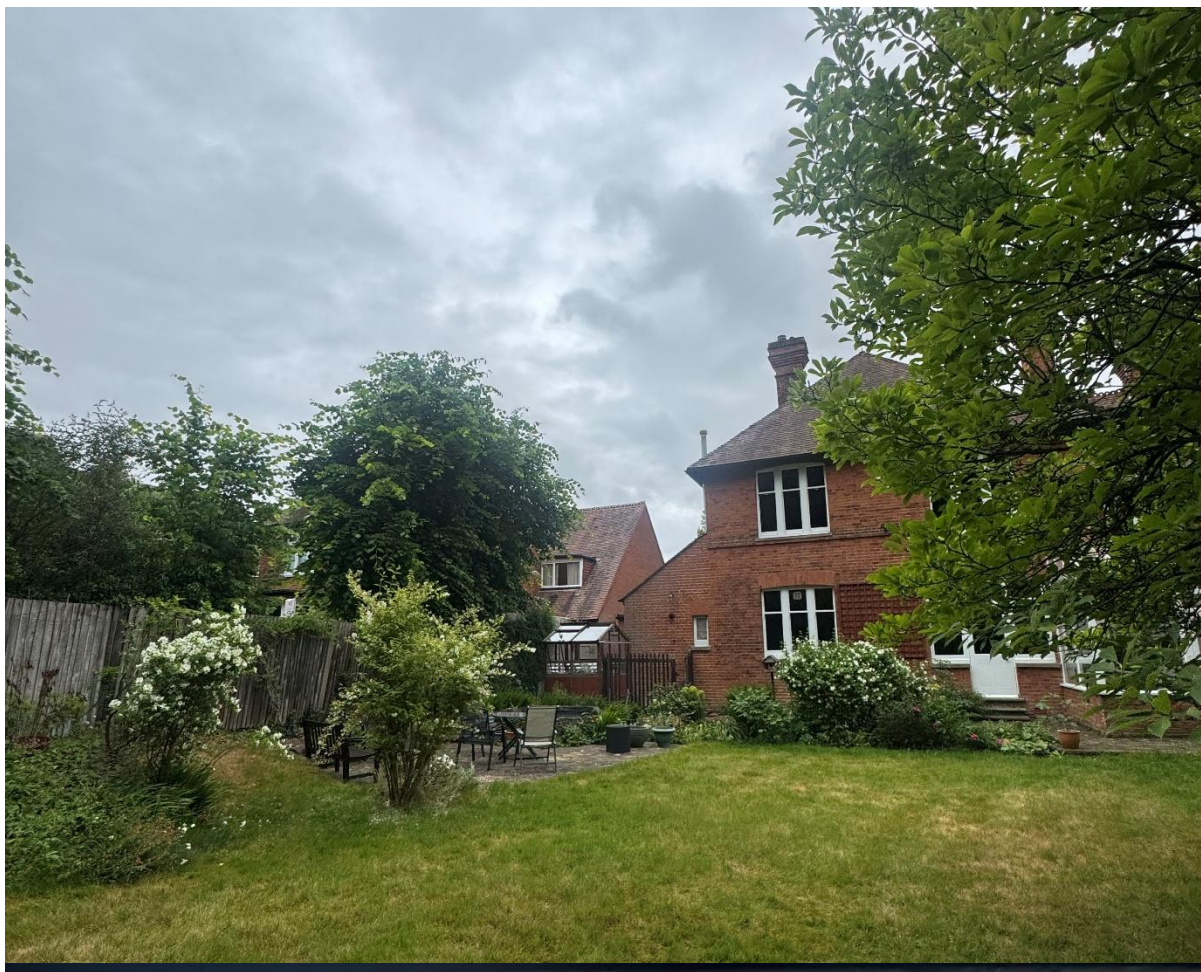
Figure 10: Rear of No. 73
