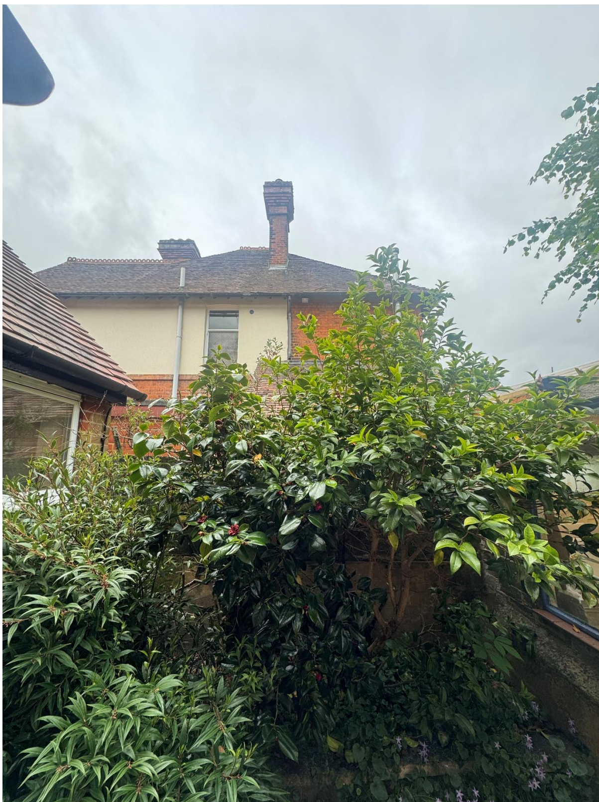
Figure 3: View towards No. 73
